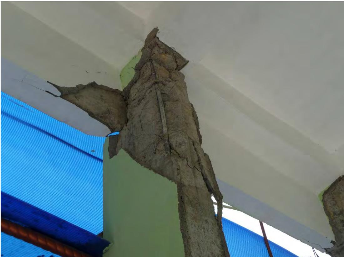
Figure 7 Missing ties in column/joint
