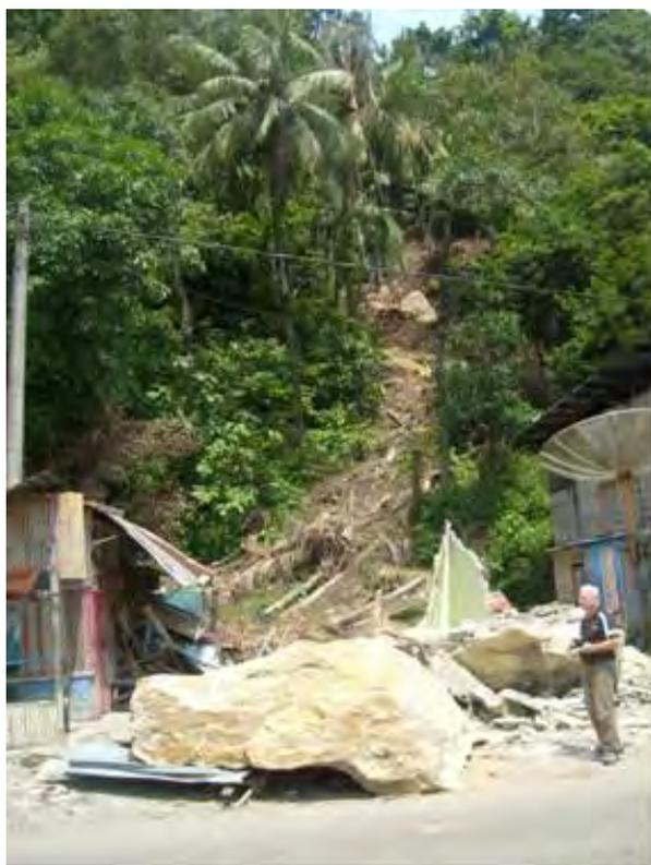
**Figure 3.7:** *Rock fall from the escarpment behind the port (Teluk Bayur)*
