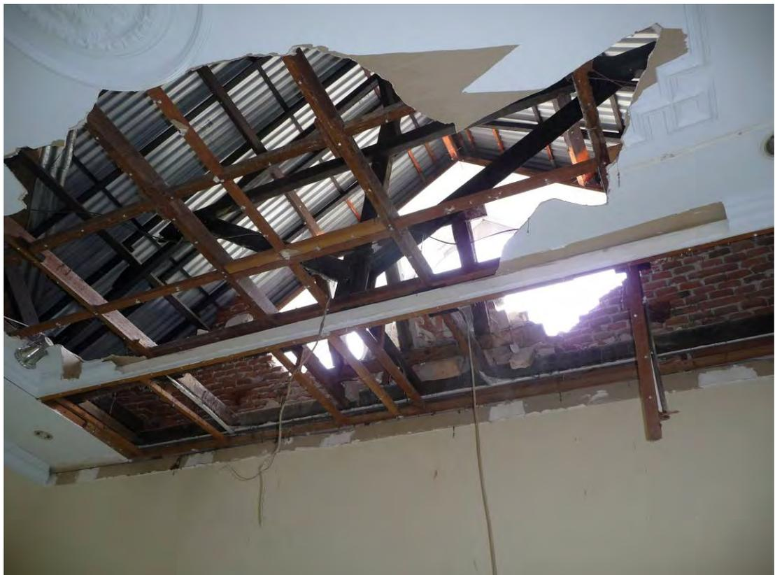
Figure 9 Failed Gable Wall
