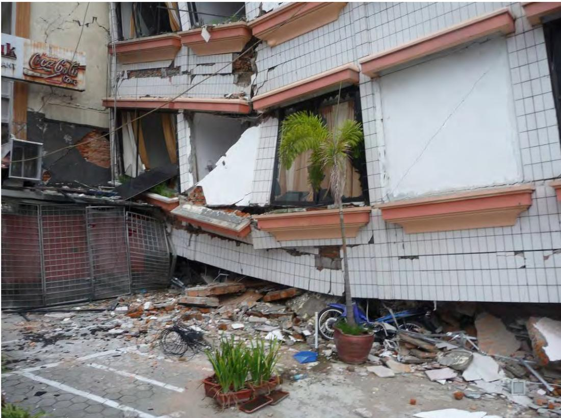
Figure 19 Soft Storey (commercial shop-front) Ground Floor Collapse
