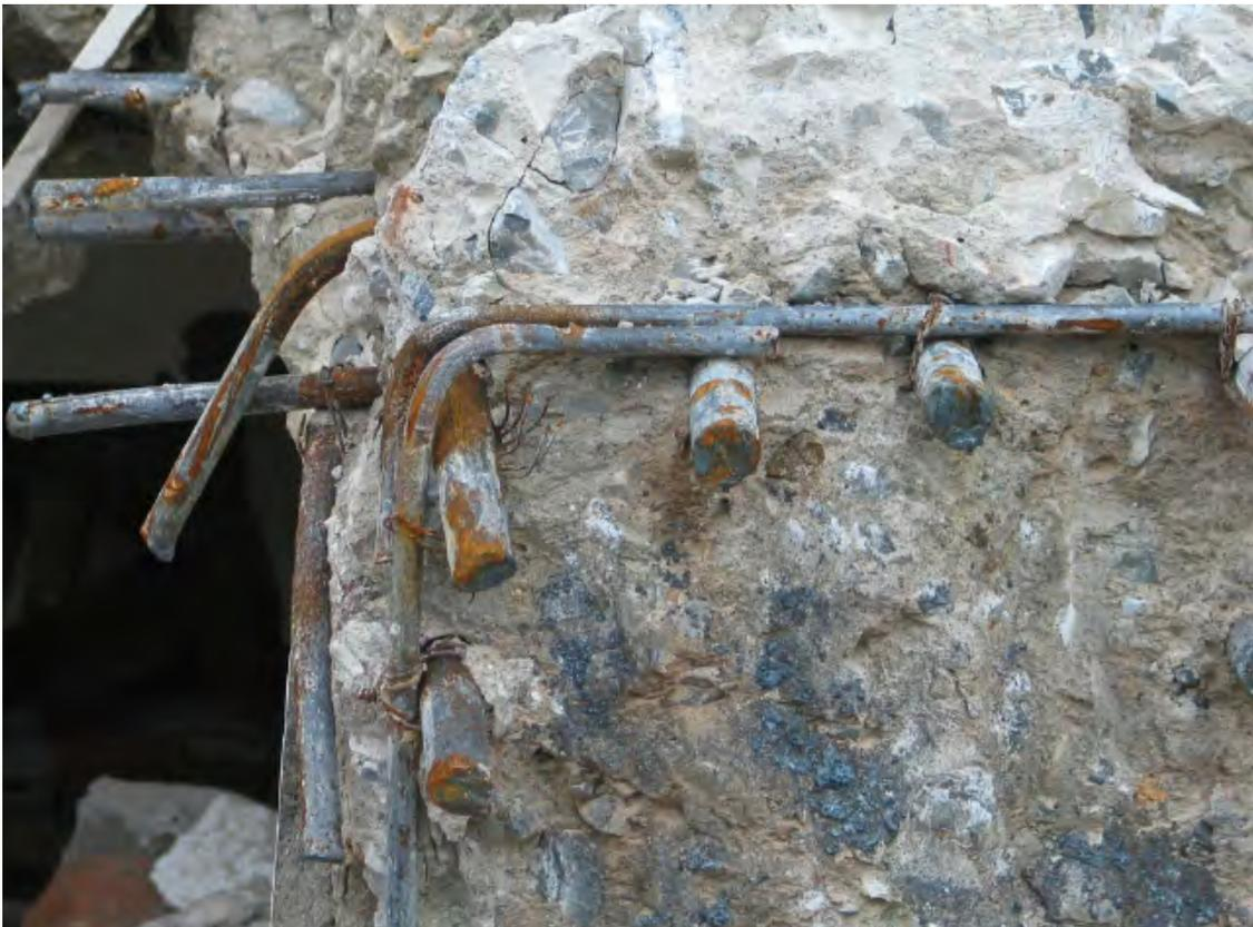
Figure 5 Poor reinforcement detailing
