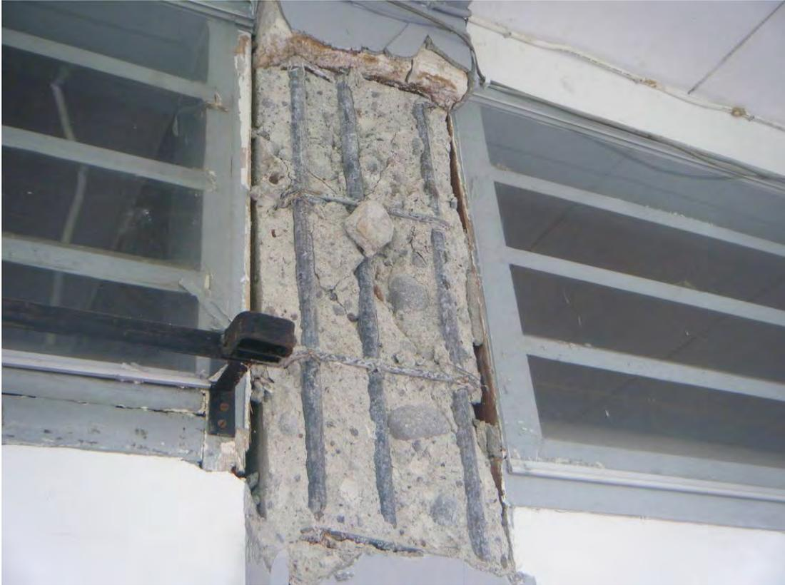
Figure 10 Poor aggregates/concrete
