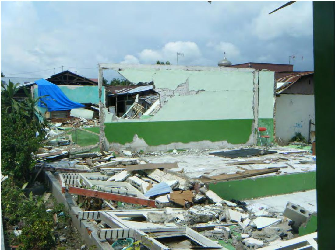
Figure 14 Collapsed school (single storey)
