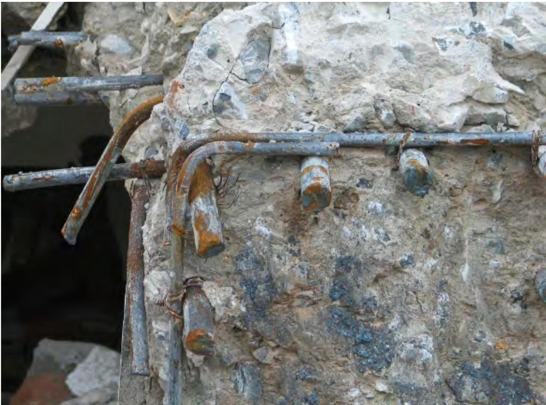
Figure 5 Poor reinforcement detailing
