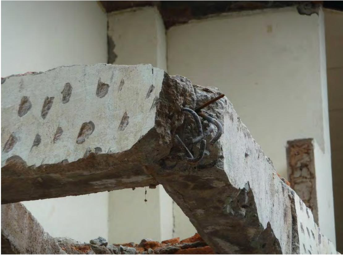
Figure 4 Poor reinforcement detailing
