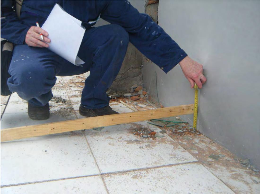
Figure 24 Liquefaction caused heavier buildings to sink
