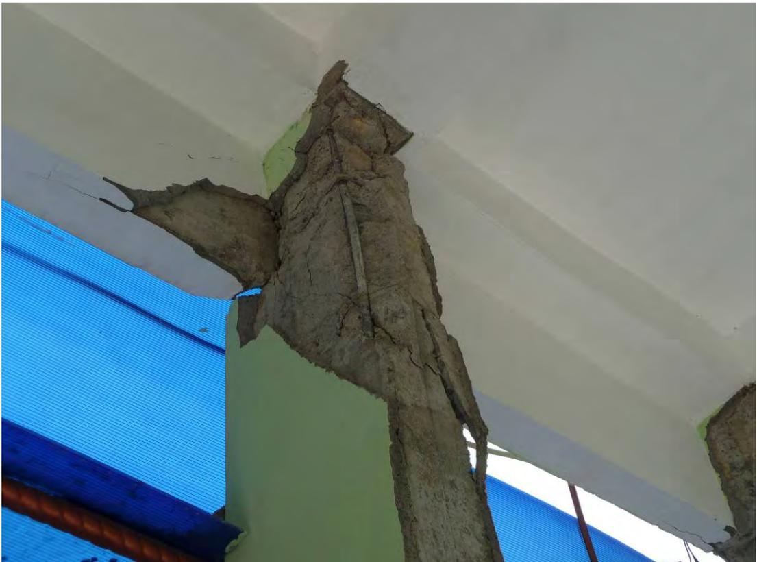
Figure 7 Missing ties in column/joint
