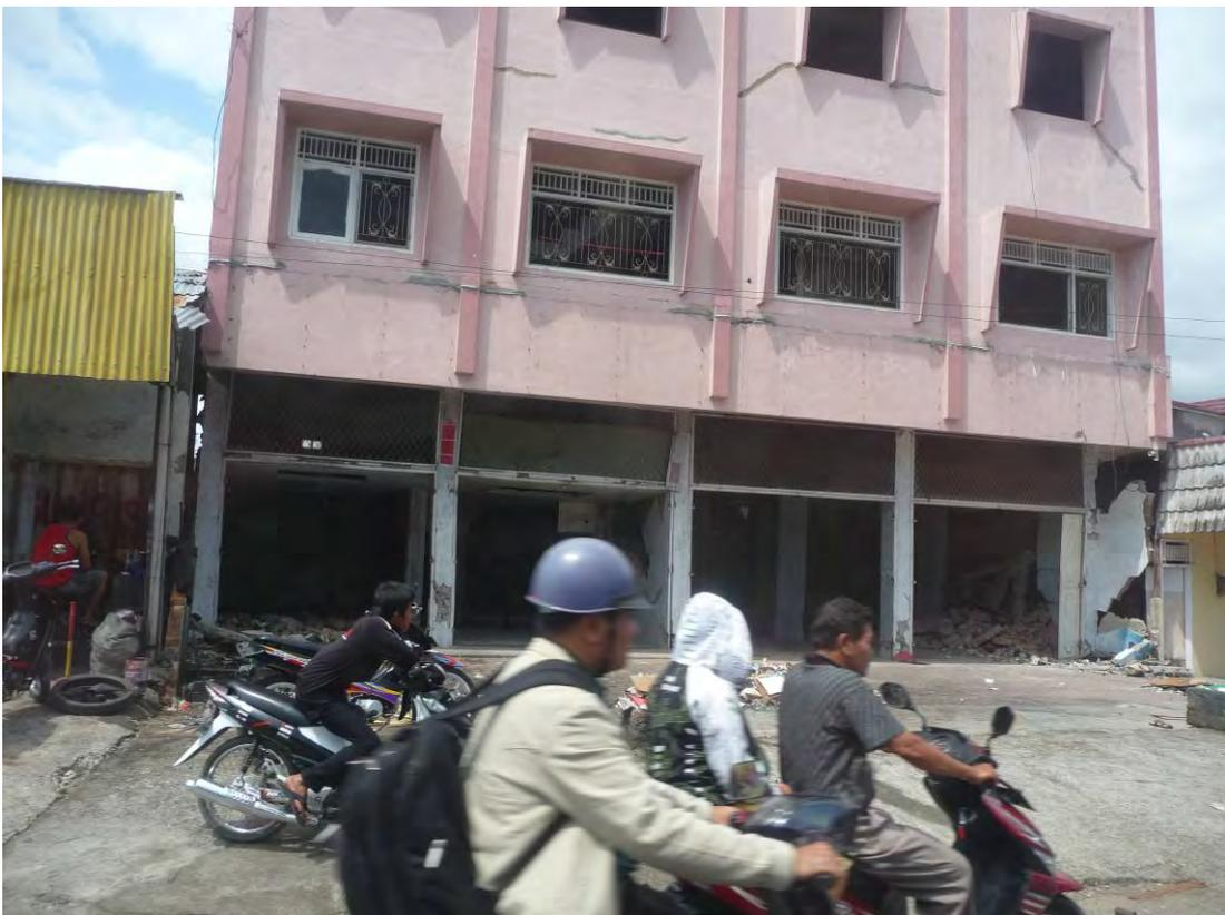
Figure 21 Another soft storey building near collapse
