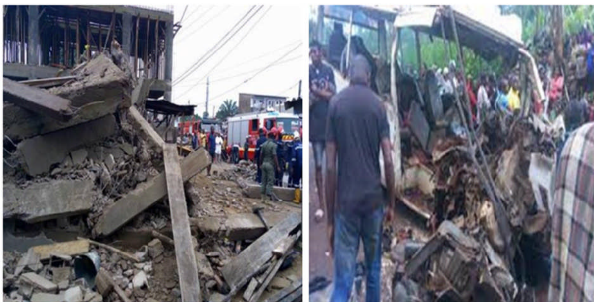
1) Collapse of a building in Douala – Ndogbom in 2016 (left); 2) Road accident in June 2019 at the “col Batié” in the West Region (right).
