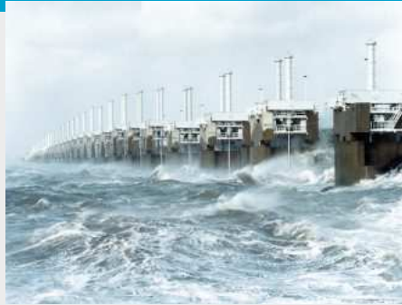
Safety, protection against flooding
