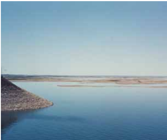
Views of the Falcon dam, State of Tamaulipas
