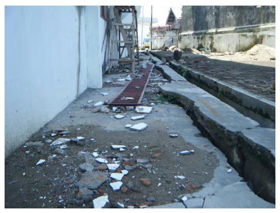
Figure 22 Settlement due to liquefaction (note sand forced up through cracks in concrete)
