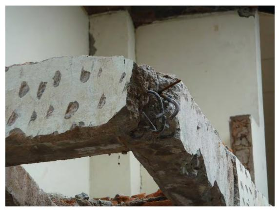
Figure 4 Poor reinforcement detailing
