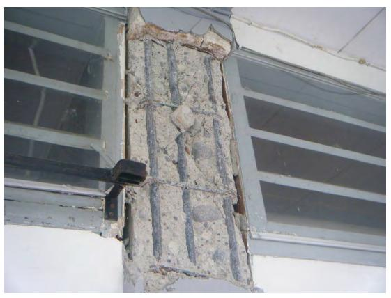
Figure 10 Poor aggregates/concrete
