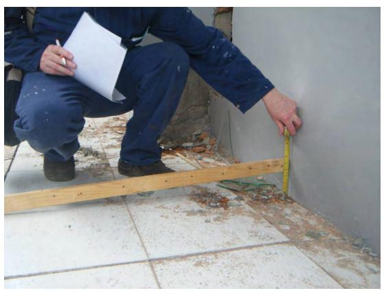
Figure 24 Liquefaction caused heavier buildings to sink
