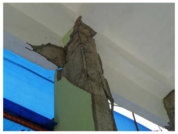
Figure 7 Missing ties in column/joint
