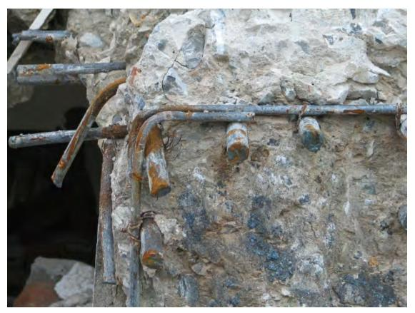
Figure 5 Poor reinforcement detailing
