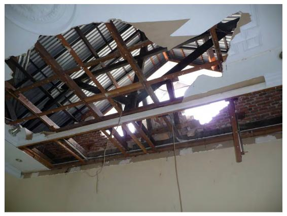
Figure 9 Failed Gable Wall
