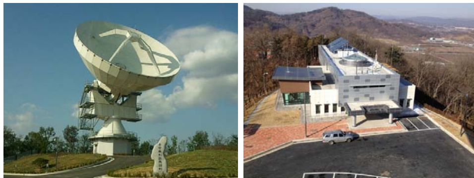
Figure 2.Geodetic VLBI station with facilities in Sejong city
