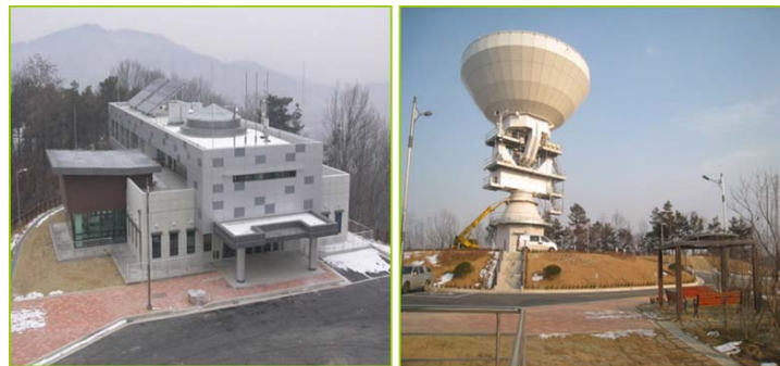
Figure 2. Geodetic VLBI station with facilities in Sejong city
