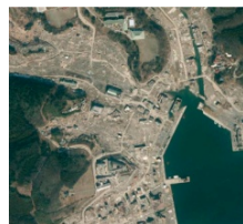
After earthquake disaster (image taken on March 19, 2011)
